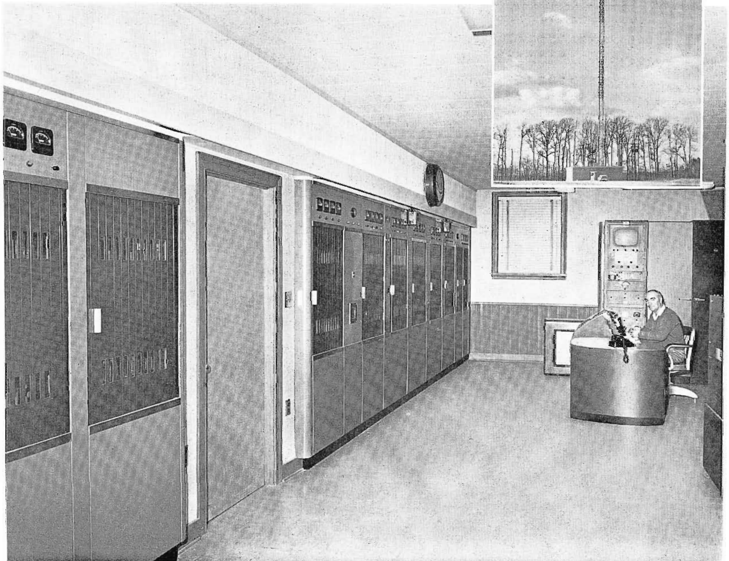
FIG. 1. WBOC-TV's TTU-12A Transmitter as it appears today. The 600-foot tower and antenna are shown in the inset.
