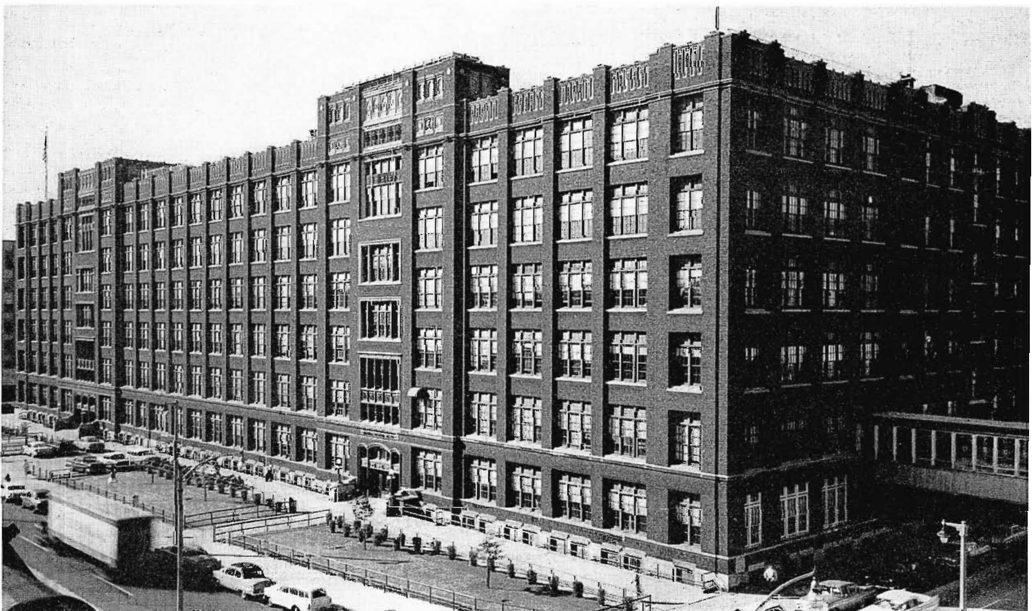
FIG. 3B. Milwaukee Vocational and Adult Schools. To the right is second floor overpass leading to the Tech building (Fig. 3A). The five divisions of the Vocational School last year had over 30,000 students enrolled in various courses.
