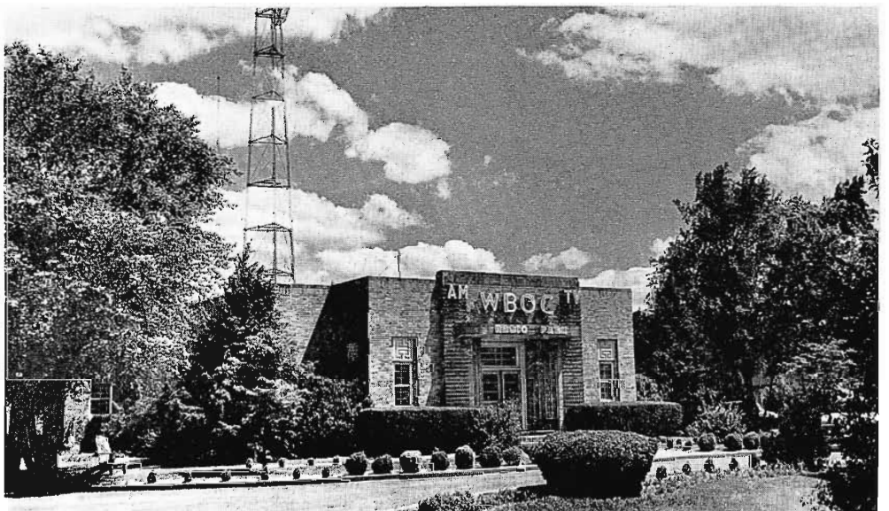
FIG. 17. Radio-TV Park, Salisbury, Md. The original building, erected during 1940, has experienced no change in silhouette despite three major expansions to include all station facilities except for the TV transmitter.
